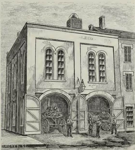
SOUTH HIGH STREET ENGINE HOUSE.
